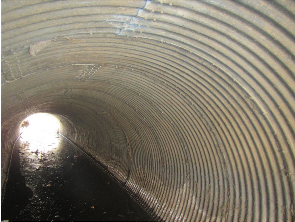
Picture 2 – Inside of pipe
